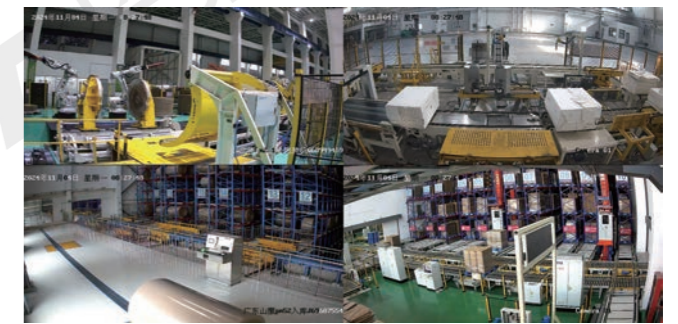
现场监控大屏
